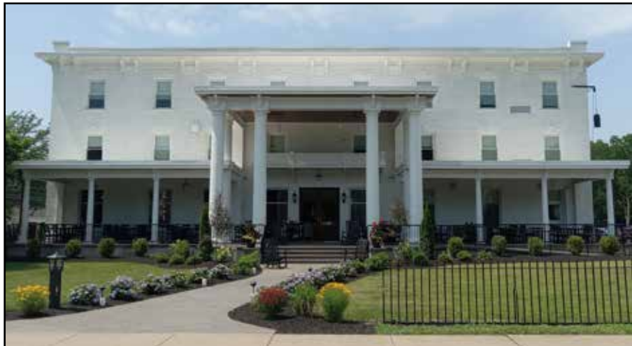
The White Inn, located at 52 E. Main Rd. in Fredonia, held its grand opening and ribbon cutting on Thursday, June 26. The historic building opened following a multimillion dollar renovation effort by developer Steve St. George, along with business partner and executive chef Devin Jones.
