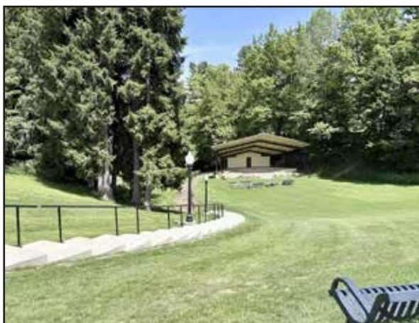
The completed stairs with railings and lights.
